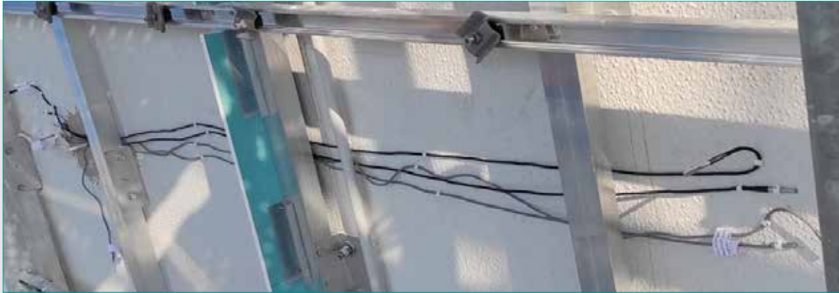
Fig. 7 - Installation of temperature sensor probes inside the ventilated façade cavity.
